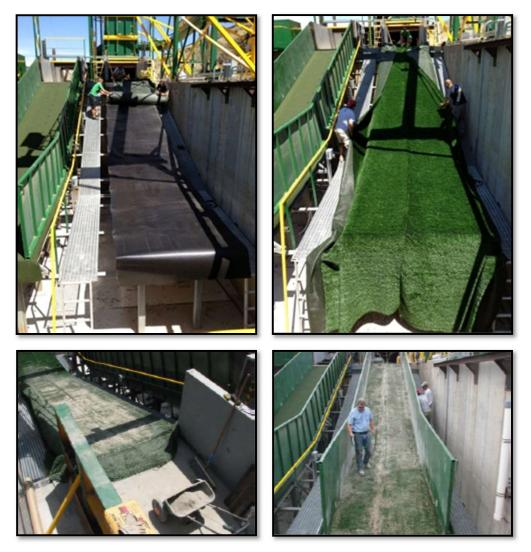
Figure 3. HydroTurf® System Installation
